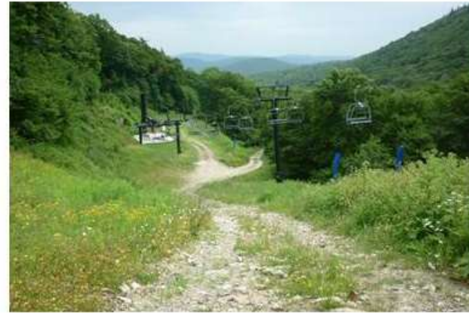
5. View downstream along maintenance roads to bottom of Canyon Quad lift.
