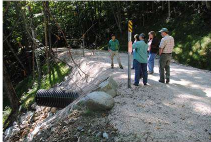
2. View downhill, same culvert site as photo 1.
