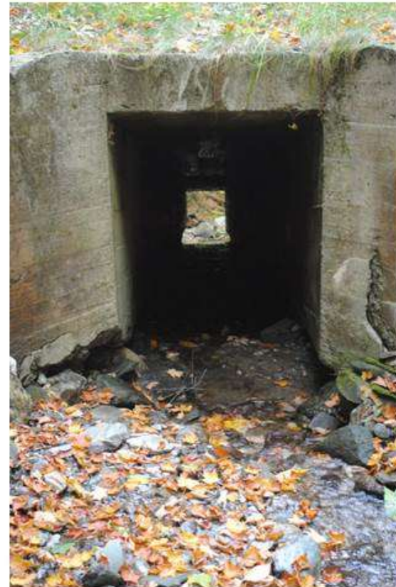
2. View downstream through box culvert.
