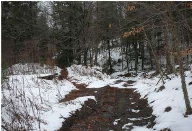
7. View downhill from photo 6; road drainage runs off to nearby stream
