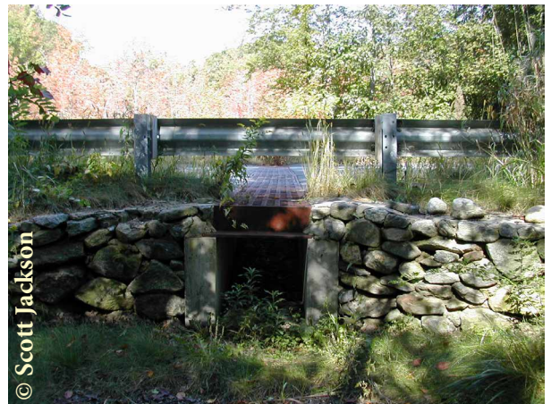
Salamander tunnels provide safe passage across busy roads.
